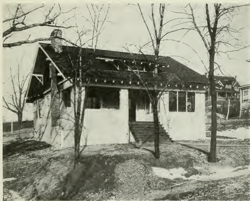
FIGS. 35 AND 36.—REINFORCED CONCRETE BUNGALOWS, AT CARNEGIE, PA., U.S.A.
